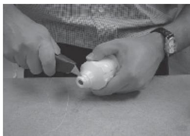
1. Cut boot at first line for cable greater than 10/3 (or greater than 5/8" Dia.).
